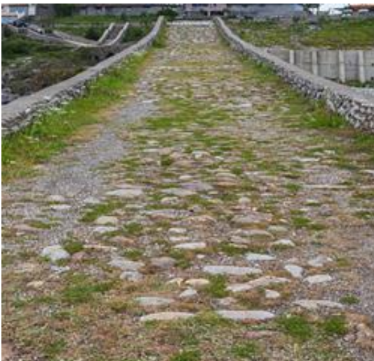
FIG. 7. The Bridge of Mesi paving with full gravel
