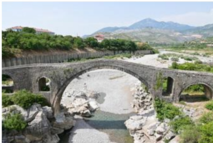
FIG. 3. The Bridge of Mesi, with lateral holes.
