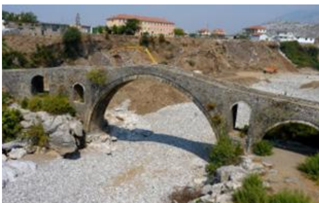
FIG. 4.A,B. The Bridge of Mesi, built during the Ottoman period, around 1770, by a local Pasha, on the Kiri River. The bridge is 120m long, 3.4m meters wide, 12.5 meters high with 13 arches and represents one of the longest Ottoman bridges in the region.
