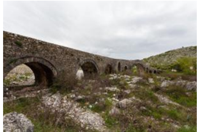
FIG. 6. The Bridge of Mesi, presentation of the stone façade
