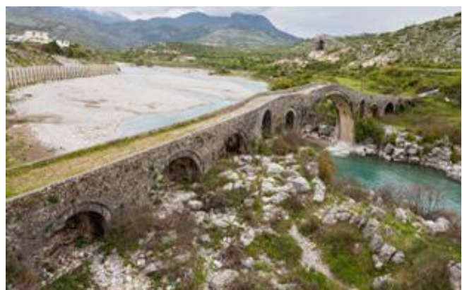
FIG. 4.A,B. The Bridge of Mesi, built during the Ottoman period, around 1770, by a local Pasha, on the Kiri River. The bridge is 120m long, 3.4m meters wide, 12.5 meters high with 13 arches and represents one of the longest Ottoman bridges in the region.
