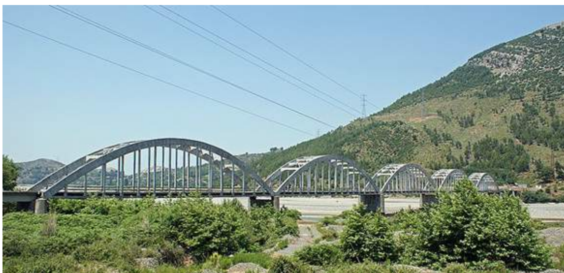
FIG. 2 Picture of the Zogu Bridge, 2011
