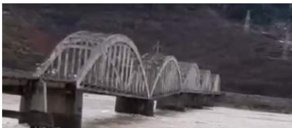
FIG. 5 – The first three spans of the Zogu bridge now showing the exposed piling and some additional supporting scaffolding
