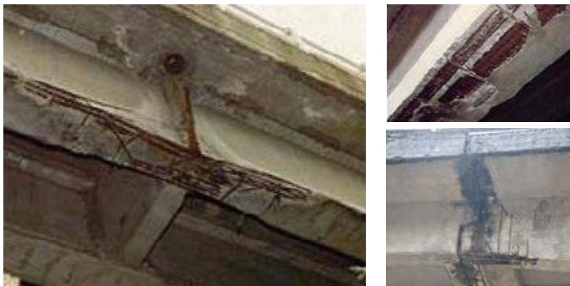
FIG.1 - Example of damage and decay in r.c. structural element - RAM Project, Road Asset Management– Main Inspection Handbook (Anas- Italian FS Group)
