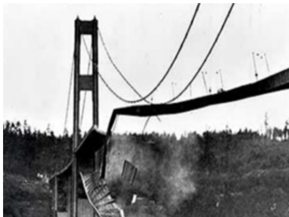
FIG.12 – November 1940. Tacoma Bridge collapsed for the vibrations induced by the wind
