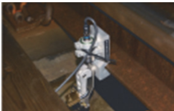
FIG.10 - An energy harvester prototype, installed on the Old Lidingö Bridge (Rosengren et al., 2017)
