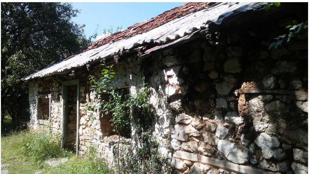
PIC. 5: Apartment in Stëblevë, Librazhd - inhabited until the beginning of 1992. Photographed in 2019.
